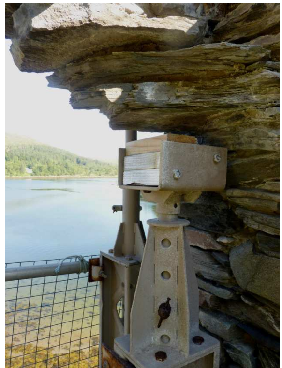
2014, detail, showing failed loose propping & missing packing etc.
